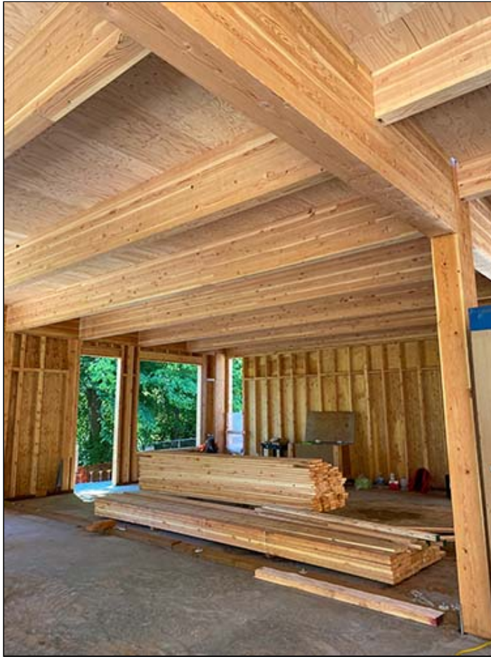
Mass plywood panels and glulam beams are on full display inside the building.
