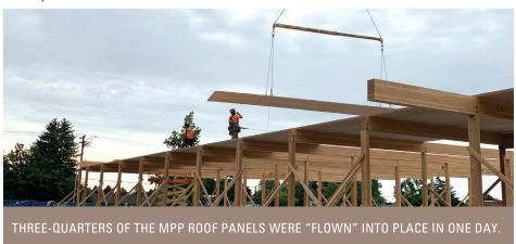
The building construction includes concrete foundations, slab on grade, steel, mass timber and conventional wood framing systems. Building with mass timber shortened the construction significantly, so the new ag complex would open in time for the upcoming school term.
