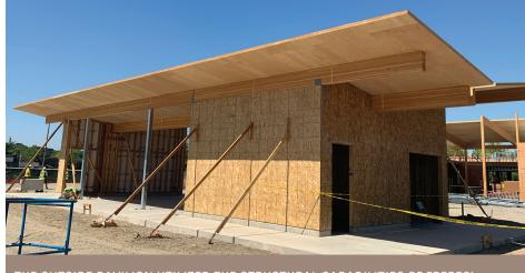
THE OUTSIDE PAVILION UTILIZED THE STRUCTURAL CAPABILITIES OF FRERES' PANELS TO ALLOW FOR EXTREME CANTILEVERS IN THE BUILDING DESIGN.
