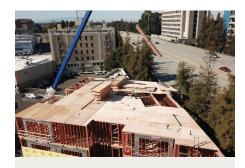
Twenty-four working days into the build, the four-story residential building stood completed. Using MPP and other prefabricated materials allowed Gurnet Point to build much faster than would have been possible with traditional stick framing materials, especially due to not needing lay-down space onsite.
