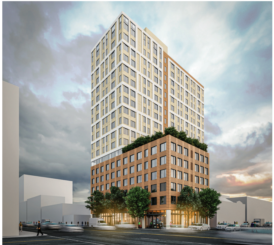
Rendering of oWOW's 19-story affordable housing project. Freres Engineered Wood's Mass Ply Panels were selected for their efficient, sustainable, easy-to-install and cost-effective attributes. Photo by oWOW
