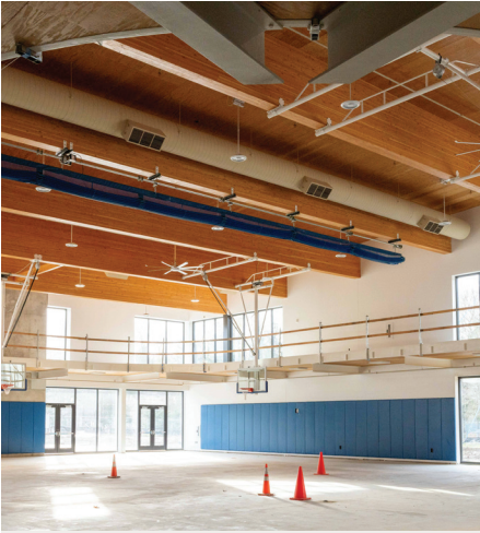
Photo provided by Carpentry Plus Inc.
