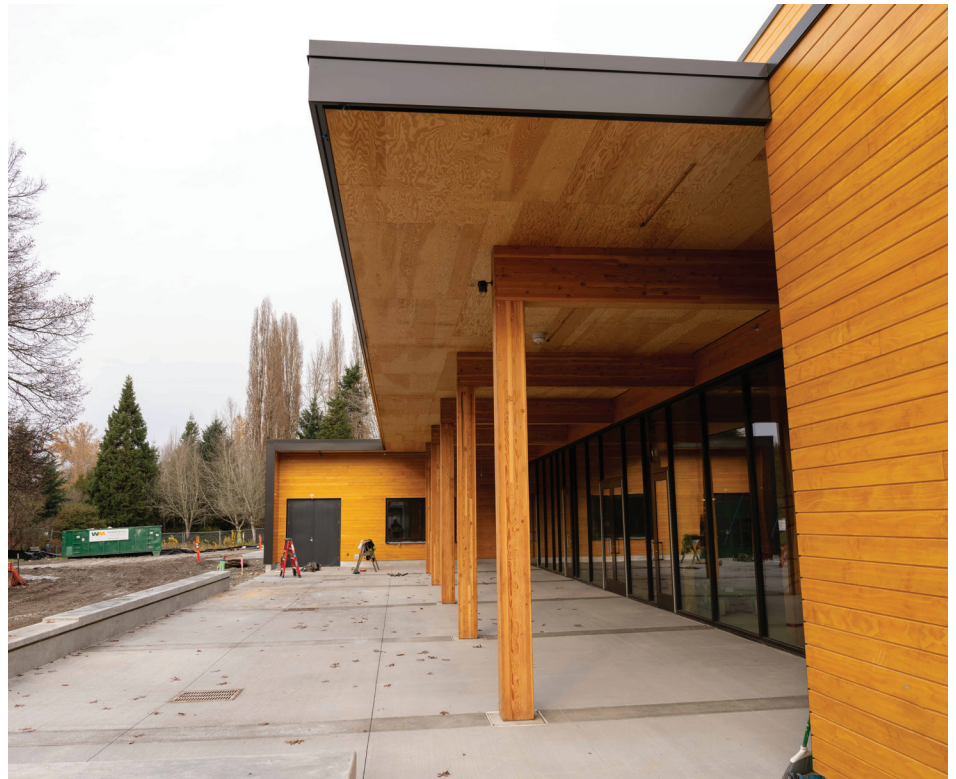
Photo provided by Carpentry Plus Inc.
