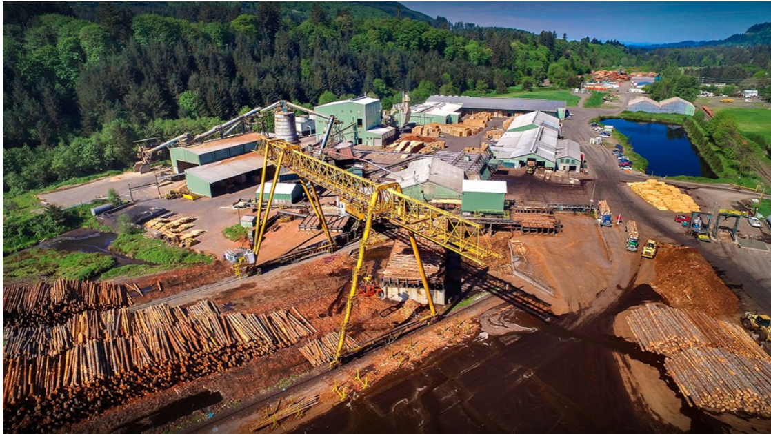
Figure 1 Freres Lumber facility at Lyons, Oregon.
