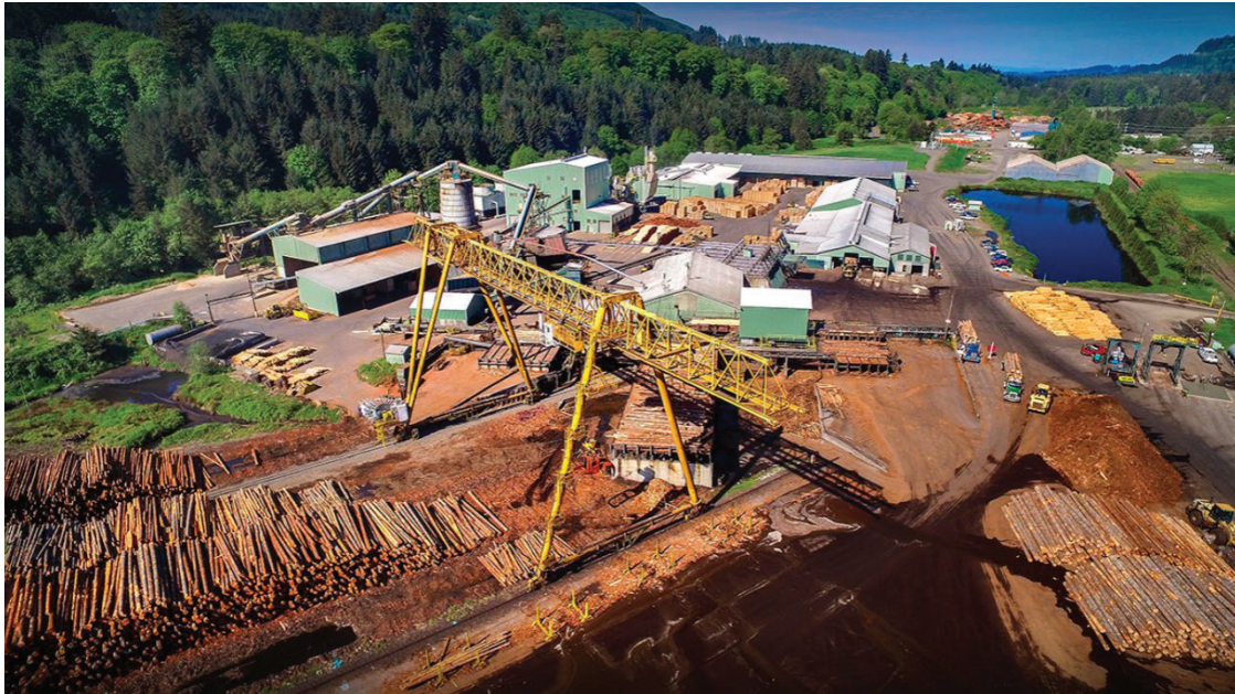
Figure 1 Freres Lumber facility at Lyons, Oregon.
